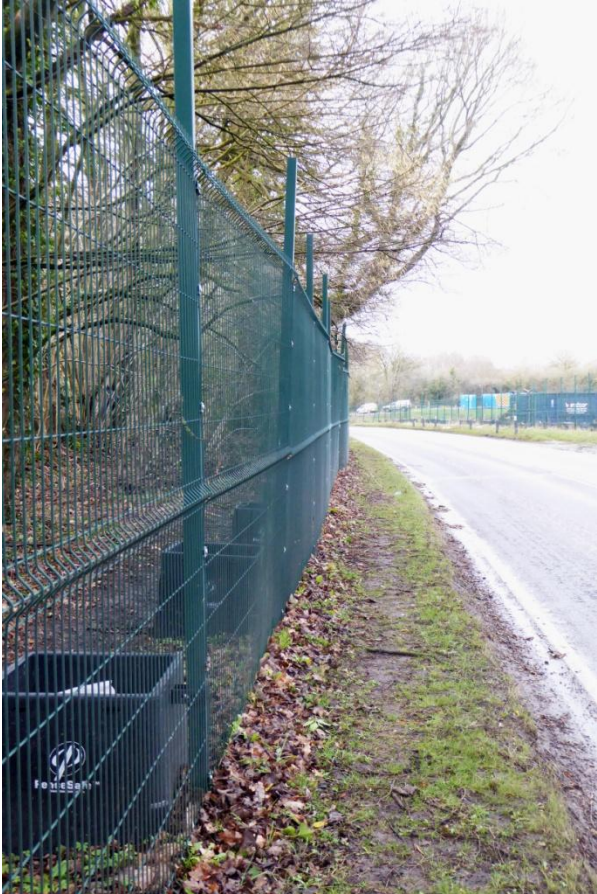
West side, showing footpath now behind the security fence, and the narrow gap remaining for pedestrians
